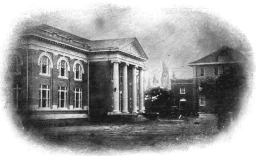
CARNEGIE LIBRARY, SHOWING PRESIDENT HULLEY'S RESIDENCE ON THE LEFT.
