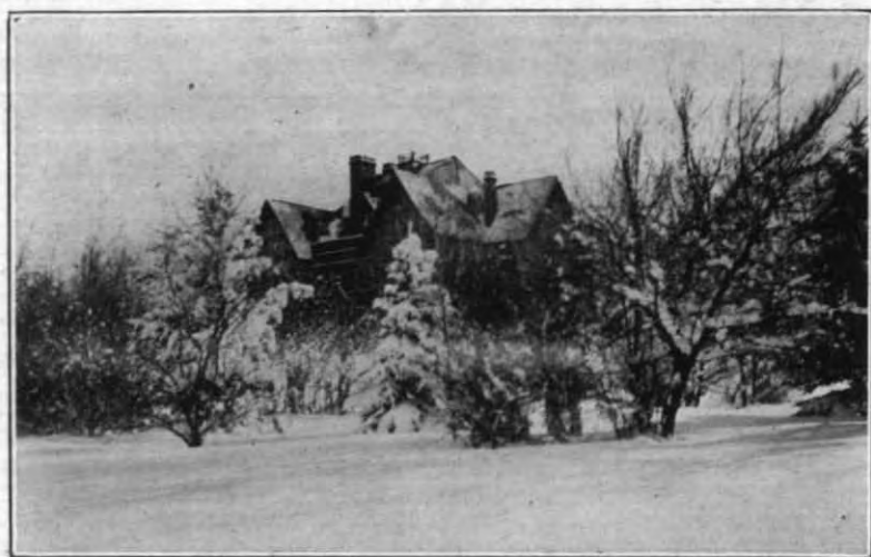
ADMINISTRATION HALL, MONTANA STATE COLLEGE
