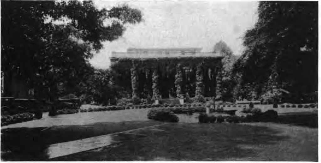
MINNIE DAVIS HALL, GIRLS' DORMITORY AT UNIVERSITY OF GEORGIA
