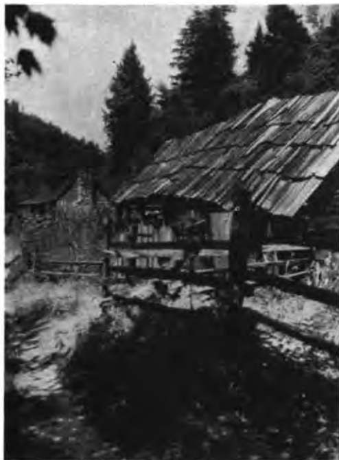
A TYPICAL COTTAGE—HAND-HEWN SHINGLES
