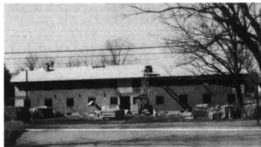
Michigan Alpha's new house under construction.
