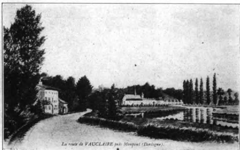
THE ROAD FROM MONPONT TO VAUCLAIRE, WELL CHEWED UP BY U. S. ARMY TRUCKS BUT NOW BEING REPLACED BY THE ENGINEERS.
