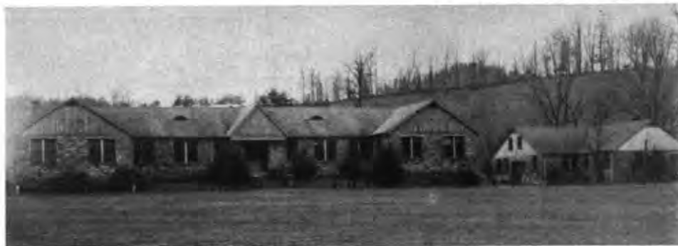
INDUSTRIAL UNIT—HIGHSCHOOL AND WEAVING BUILDING
