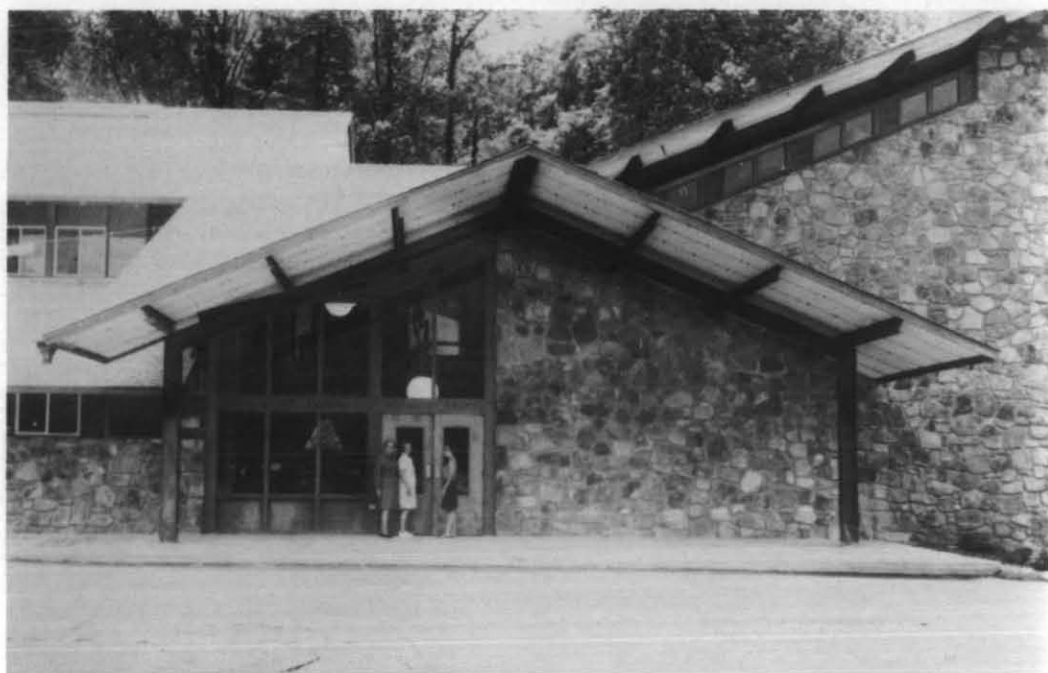
Pictured above is a close-up view of the impressive entrance to the Emma Harper Turner Building at Arrowmont
