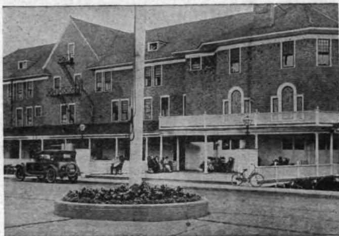
THE INN West Main Entrance
