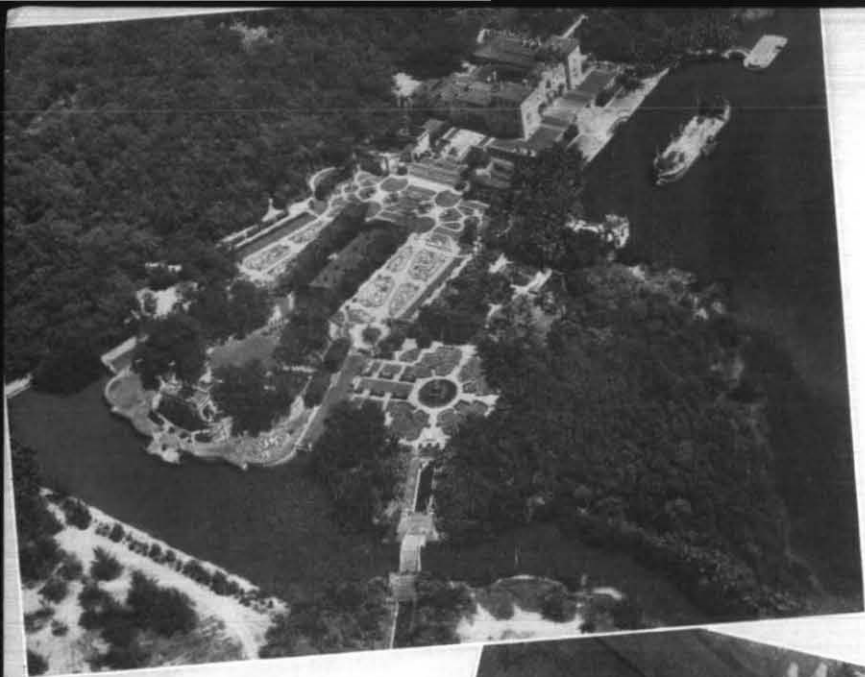
AERIAL VIEW OF VIZCAYA. Dade County Art Museum. Miami, Florida.
