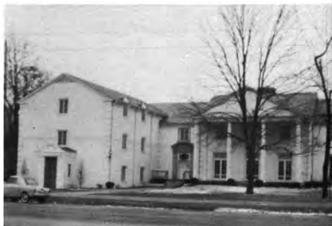
The new wing of the Indiana Gamma House
