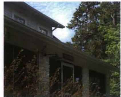
Teachers Cottage, built in 1916, is now on the National Register of Historic Places.
